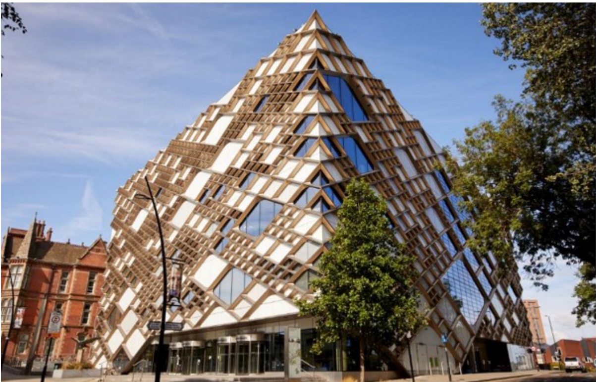
The Diamond – Engineering Department at The University of Sheffield
